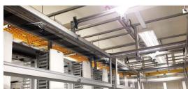
The Fire Suppression Access Ceiling is the perfect addition to any data center fire protection program. In the event of a fire, the ceiling adeptly falls away, allowing sprinklers or fire suppression agents to circulate freely.
